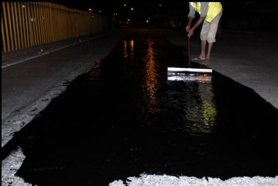
SEALKOTE application with squeeze, visible undulation of the rough surface like alligator back, final stages of wear
