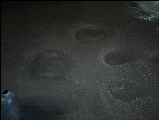
Potholes filled with water sized and shaped at the edges
