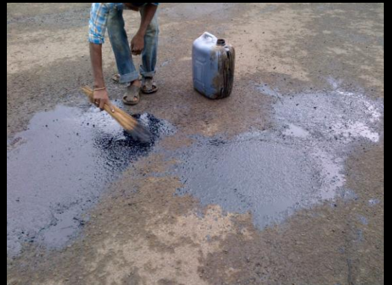
Apply SEALKOTE SB on the next day, but if the rains are heavy apply SEALKOTE SB immediately after compaction and open for traffic in 10 mins
