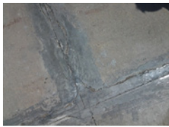
Floor joints filled with EPIGEL
