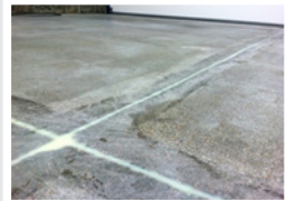
Floor joints with EPIGEL
