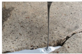
Semi rigid cracks filled with EPIGEL
