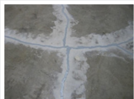
EPIKOTE LV excess grind off
