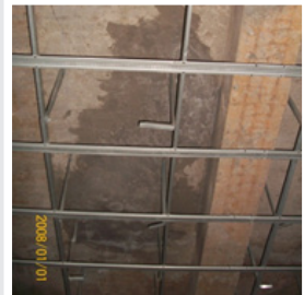
Before INCAP GROUT application
