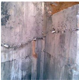
INCAP GROUT for retaining wall
