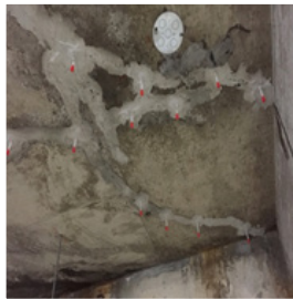
INCAP GROUT for ceiling
