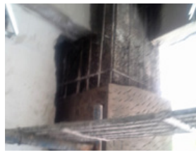
RCC jacketing stage 1
