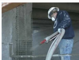
PCI 200 additive in sprayed mortar
