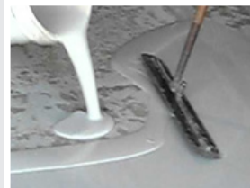
INCRETE PMR Placing stage 3
