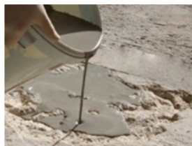
INCRETE PMR Priming stage 2
