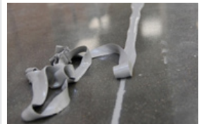
Shaving excess UREGEL off
