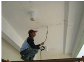
Trinity Towers Parking, Prabhadevi
