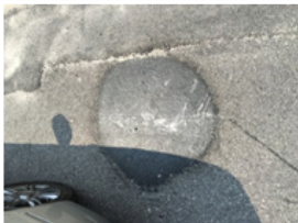
Trench Patching Seremban, Malaysia
