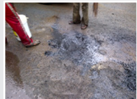
Water filled Pothole Repair PWD, Pune, India
