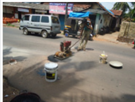
Utility Patch Repair Mangalore, India
