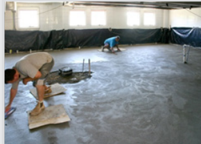
Base Preparation with Screed
