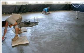
Base Preparation with Screed
